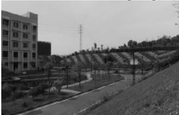
FIGURE 2 Massif slope protection greening around demonstration building
