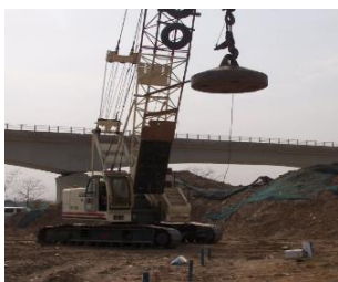
FIGURE 1 The site of dynamic compaction construction
