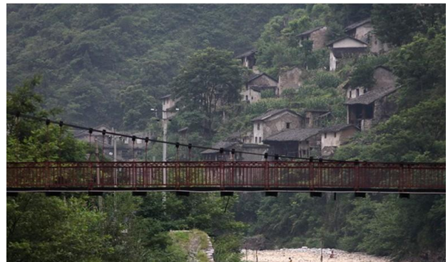
FIGURE 3 Rope Bridge at Ningchang, Wuxi country
