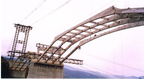
FIGURE 12 Hoisting of Rigid Frame Arch Bridge
