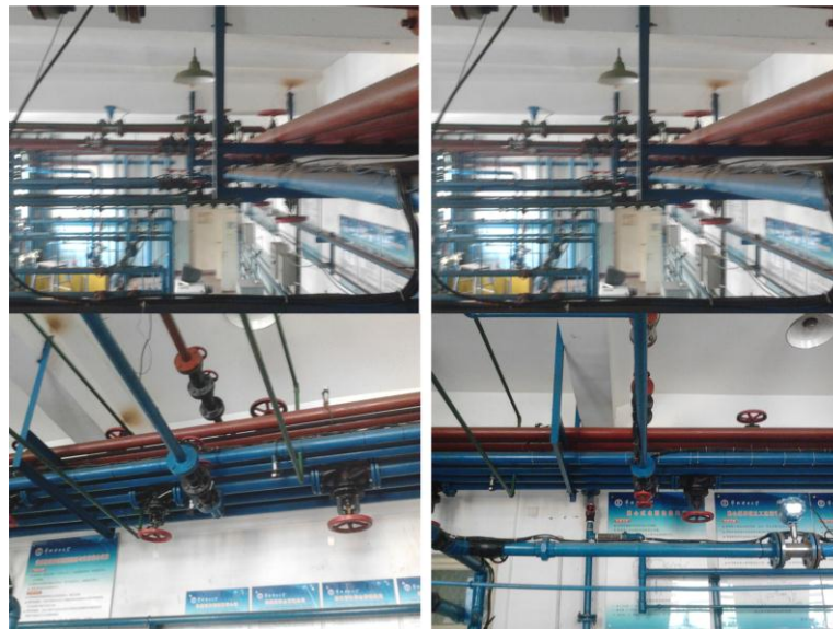
FIGURE 5 The photograph of pipe network
