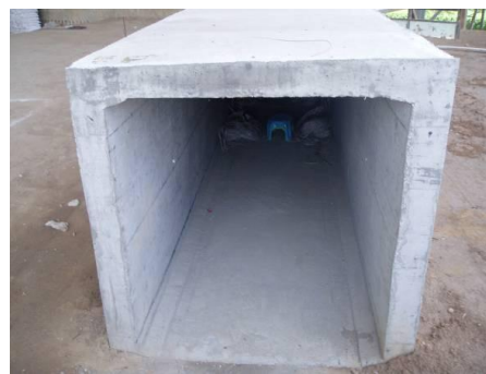
FIGURE 3 Cross Section of the Integral Box-Type Lining Structure
