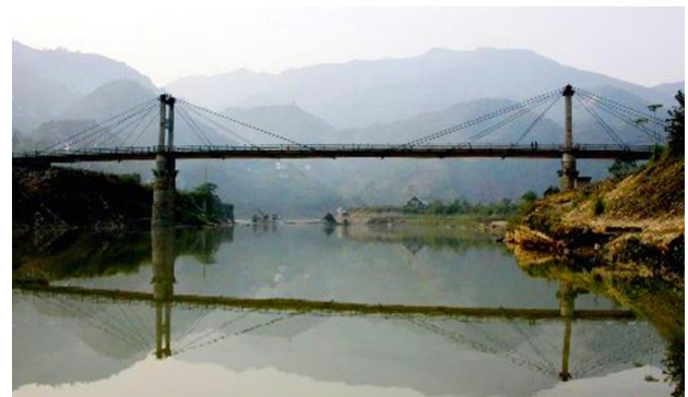
FIGURE 10 Tangxihe Cable-stayed Bridge at Yun'an, Yunyang County
