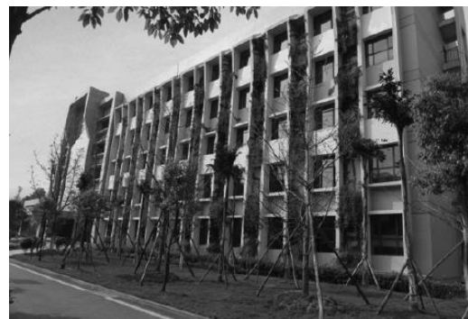
FIGURE 5 South side outer wall vertical greening
