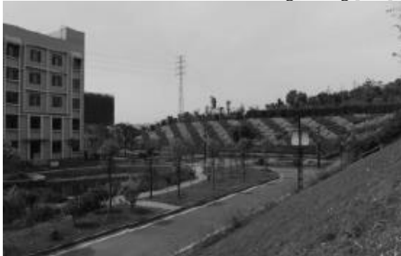
FIGURE 2 Massif slope protection greening around demonstration building
