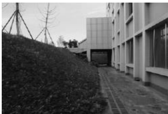
FIGURE 3 Slope greening that meet basement lighting requirement
