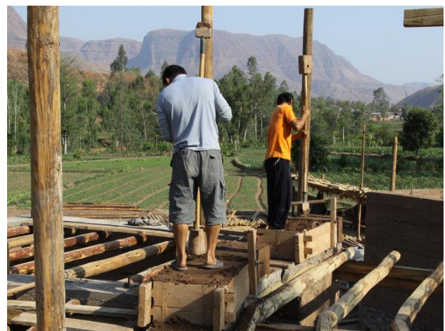
FIGURE 1 The forms and rammer used to build rammed earth walls in southern China
