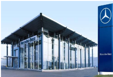
FIGURE 4 Glass curtain walls
