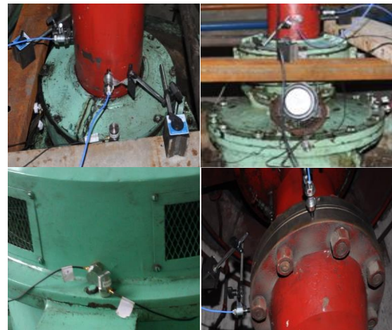
FIGURE 1 Test site arrangement
